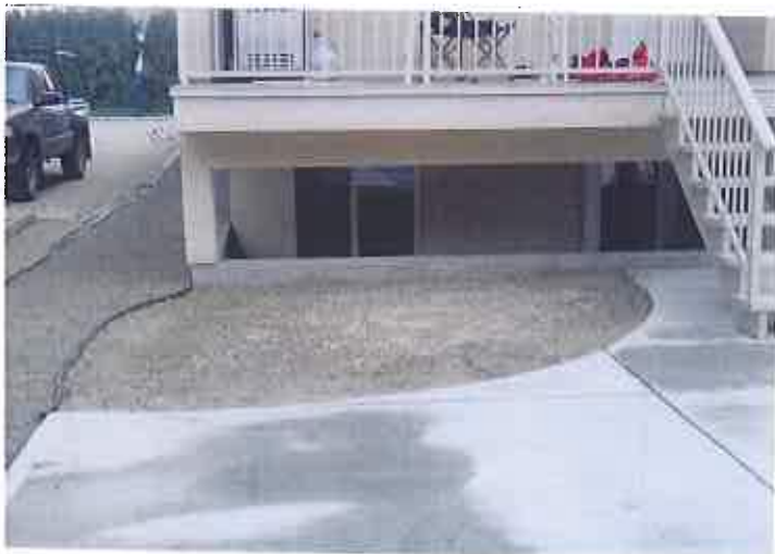
dirt area in back yard. No standing water after rain fall.
